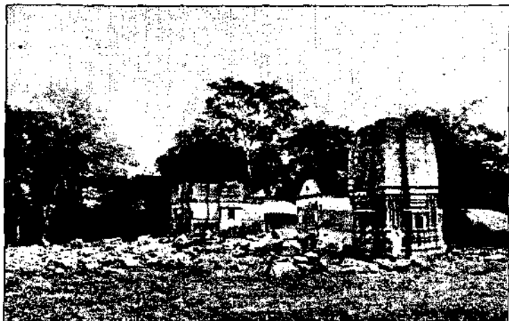
60. RUINS IN TRIVELAKK COMPOUND AT KICHING AFTER CLEARANCE OF DEBRIS, FROM S.W.
