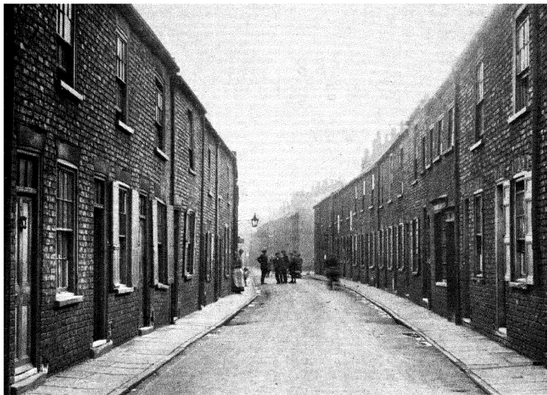
SLUM HOUSES (Before site was cleared)
