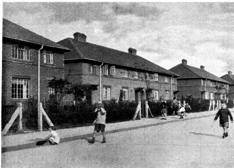
TYPICAL COUNCIL HOUSES (Category 2)
