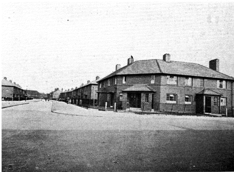
COUNCIL HOUSES BUILT ON THE SAME SITE (Occupied by tenants who previously lived in slum houses)
