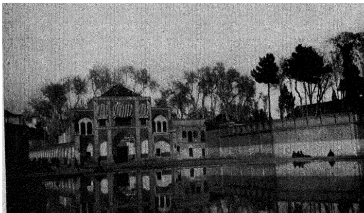
Exterior view of the Palace grounds.
