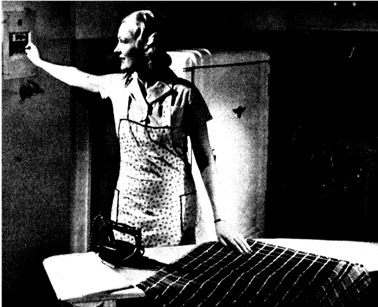
Fig. 32.5. Circuit breaker installed in a kitchen. (Courtesy Square D Co.)
