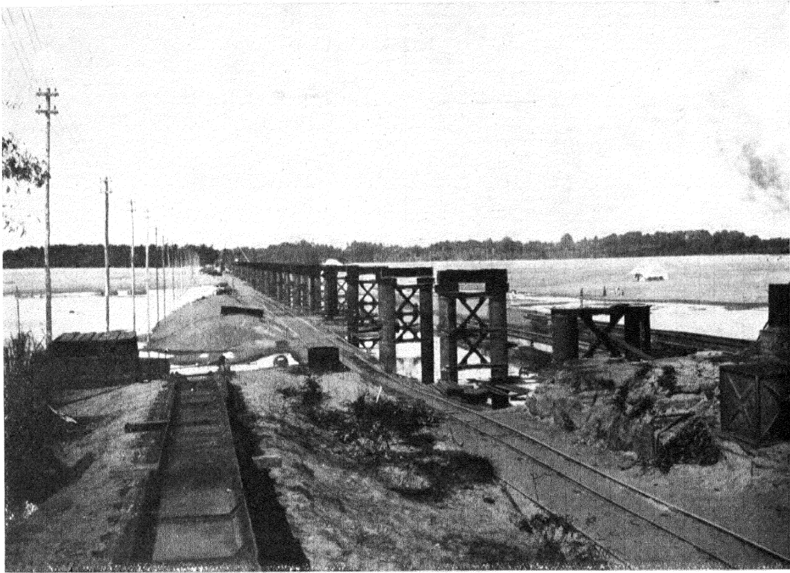
SHEWING OPERATIONS AT THE 39TH SPAN.
