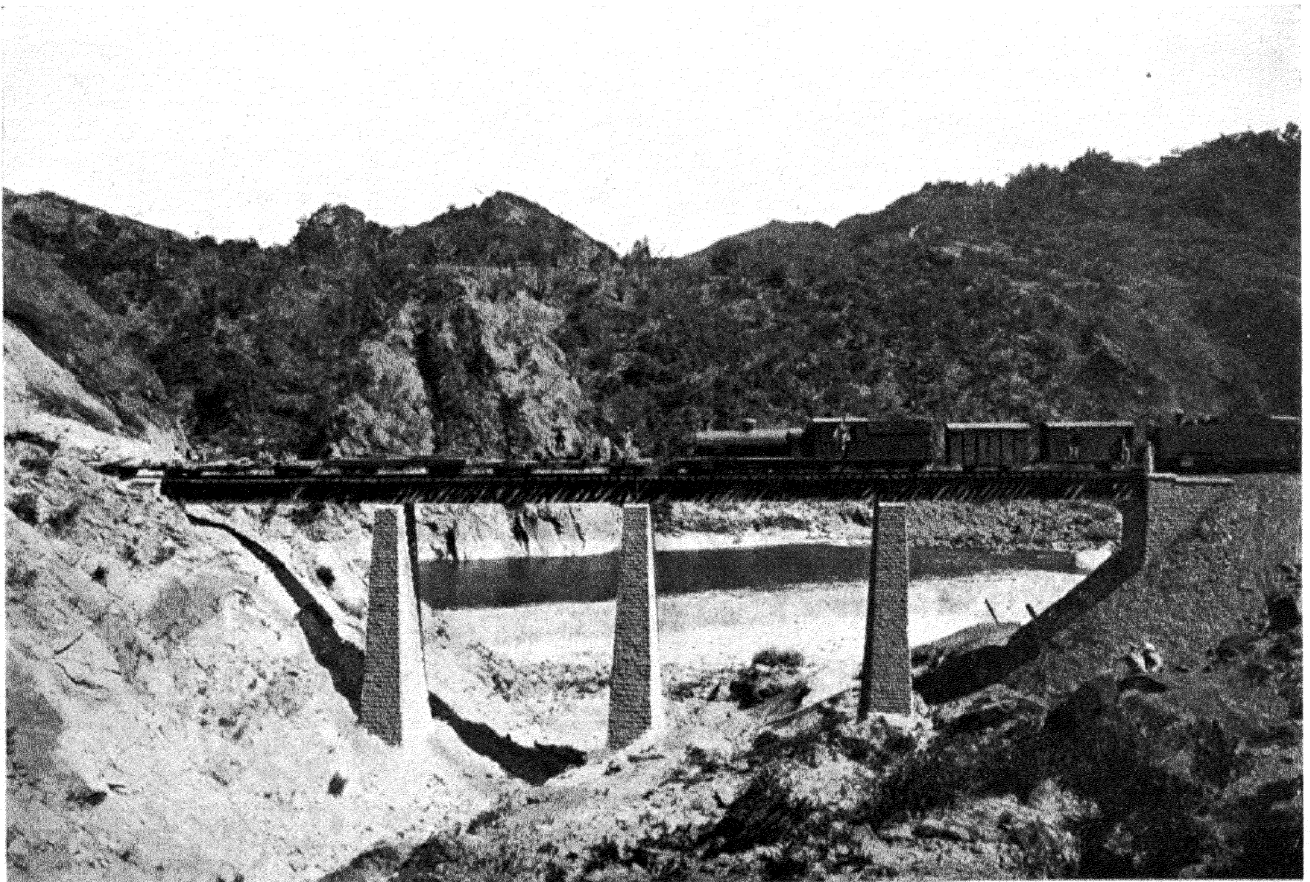
ONE OF FIVE VIADUCTS CONSTRUCTED.
