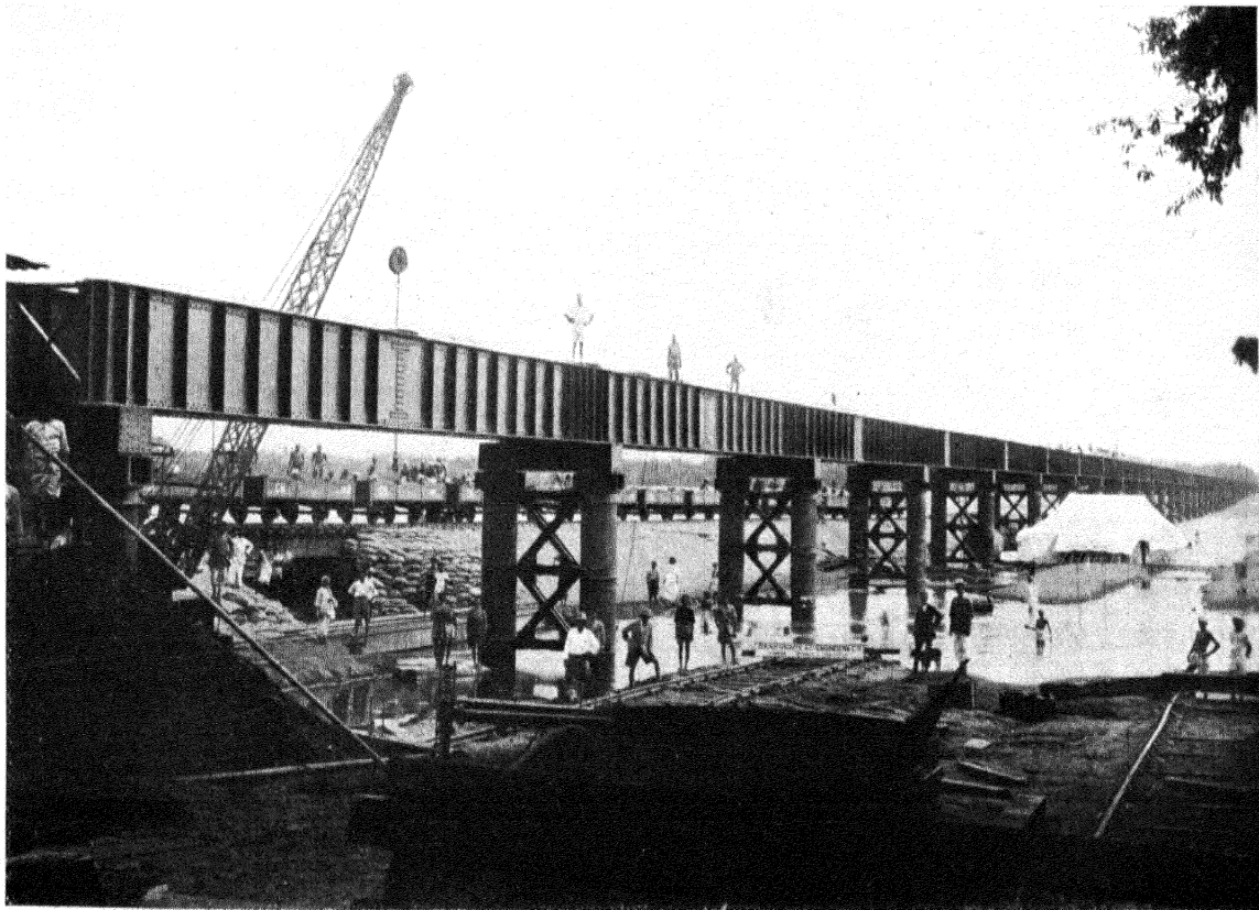
VIEW OF BRIDGE COMPLETE.
