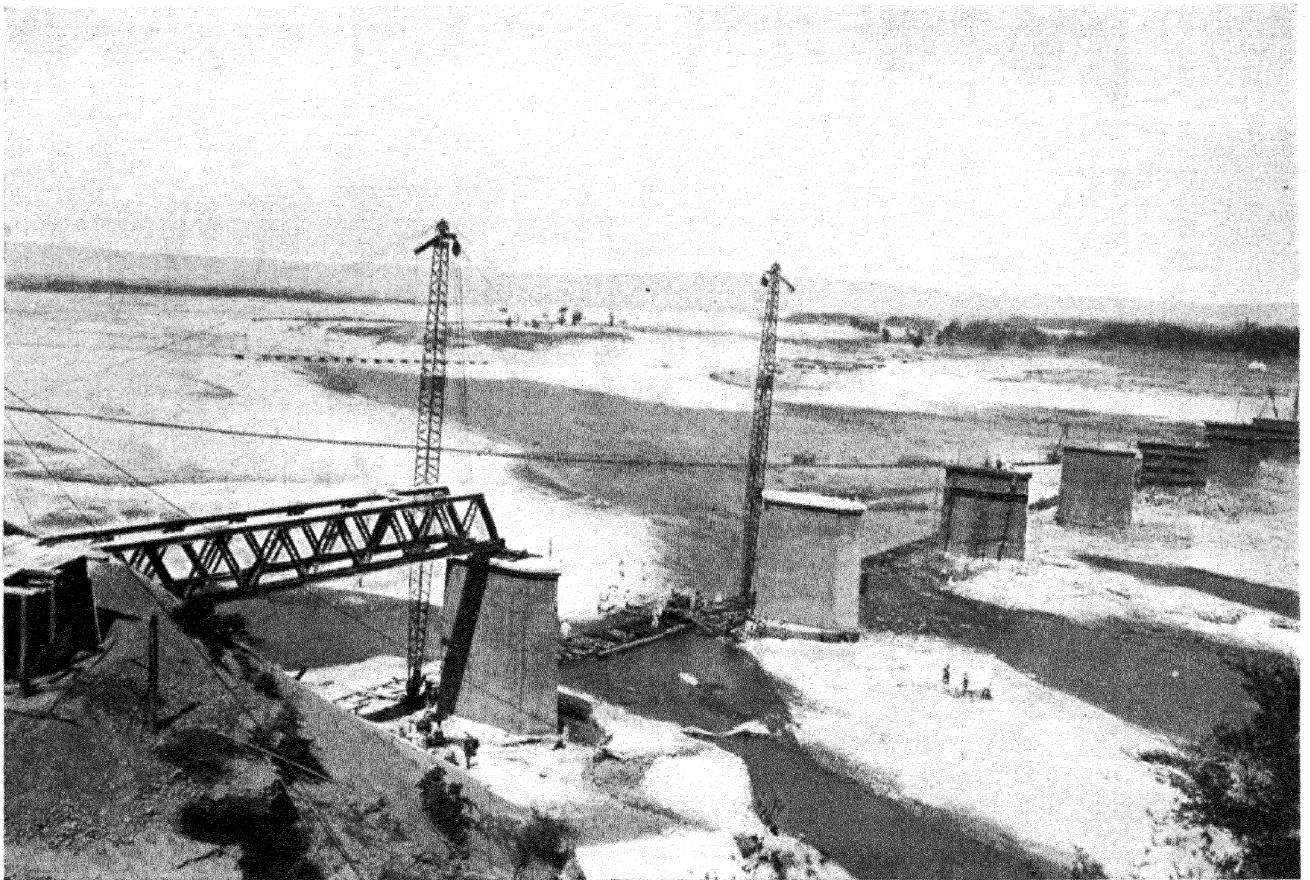
VIEW SHEWING GIRDER ERECTION IN PROGRESS AT GAJ.BRIDGE.
