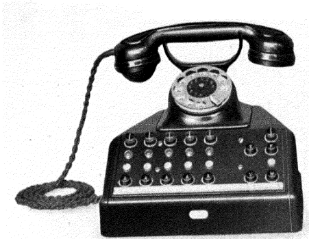
Operator's station for a Neha exchange with 5 exchange lines.
