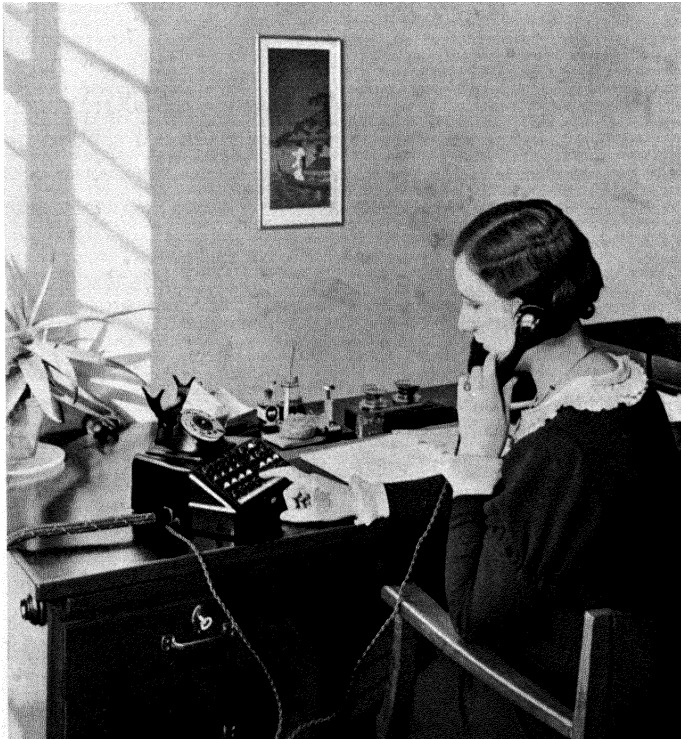
Main station of a Neha concern telephone system in the secretariat.
