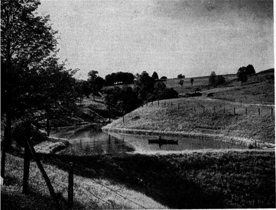
Fig. 34-11. Instead of a dangerously eroding gully, this farmer has a half-acre pond, thanks to the earth-fill dam. The pond has been stocked with fish and is now a source of food and recreation. (Courtesy of U. S. Soil Conservation Service.)
