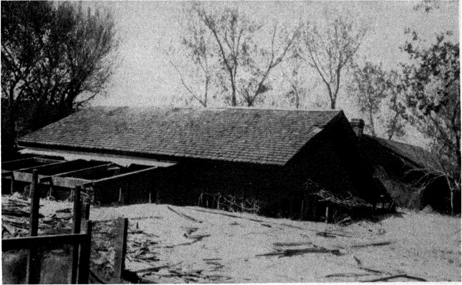
Fig. 34-7. One flood was enough to half bury this farmhouse under silt washed down from improperly farmed lands upstream. The deposit in this case was almost pure sand, valueless for farming. There was no recourse but to abandon the farm. (Courtesy of U. S. Soil Conservation Service.)
