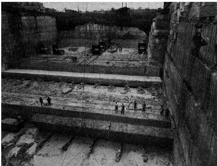
FIG. 8.—Method of turning down blocks in an Indiana limestone quarry. (Courtesy of Building Stone Association of Indiana, Inc.)
