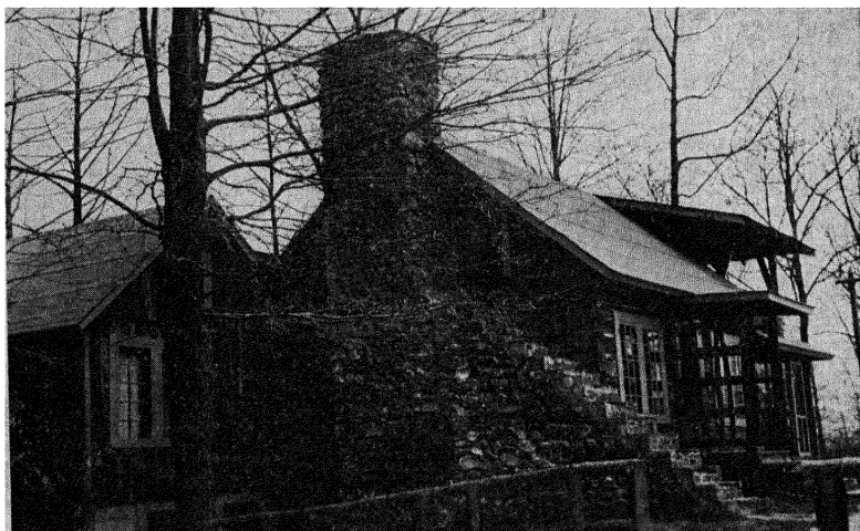
FIG. 60.—A unique type of boulder construction combining chimney with stairway. (Photo by H. Herbert Hughes.)
