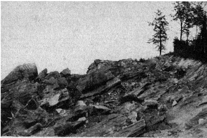
FIG. 1.—A rugged rock surface stripped by the hydraulic method.
