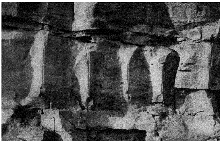
FIG. 15.—Uneven sandstone surface resulting from a break oblique to the “run.”
