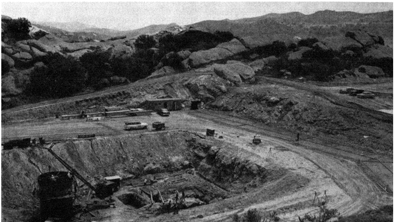
Figure 1. SRE construction in progress, May, 1955
