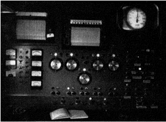
Slide 11. Photograph of control panel
