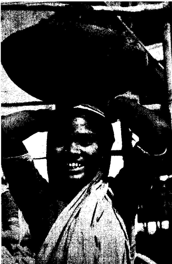
A WOMAN LABOURER CARRYING CEMENT FOR THE BUILDING OF A HOSPITAL
