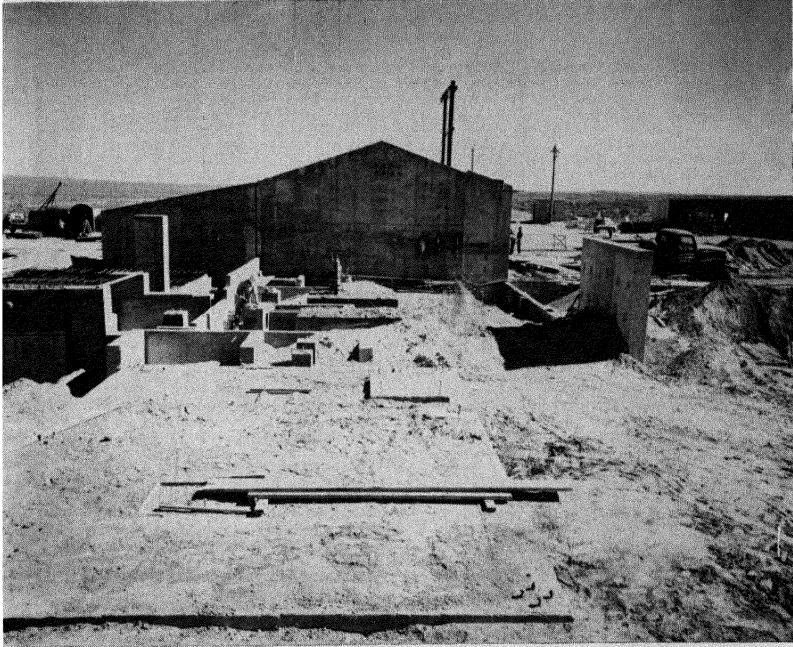
Fig. 7-33. Concrete shielding wall between the control room and the power area.
