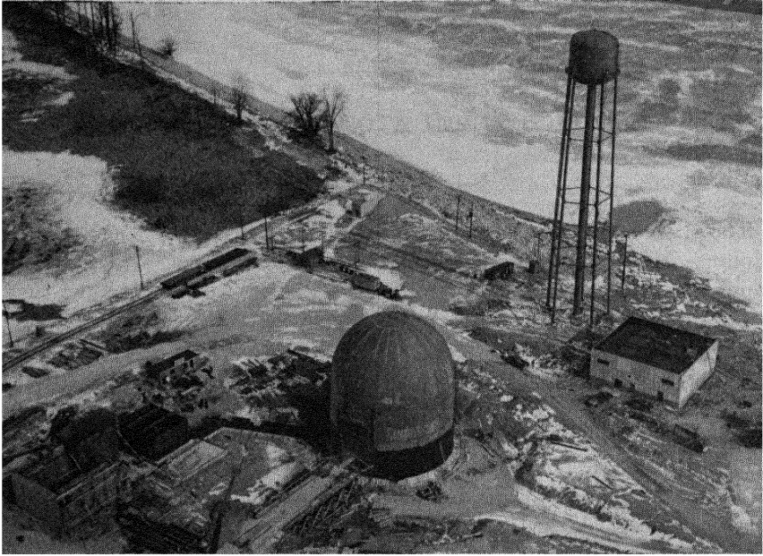
FIG. 4-1. General view of site for Enrico Fermi Atomic Power Plant.
