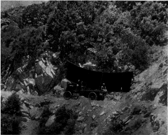
Fig. 7. Section of a steel girder for dome covering the 100-inch telescope, on its way up Mount Wilson.
