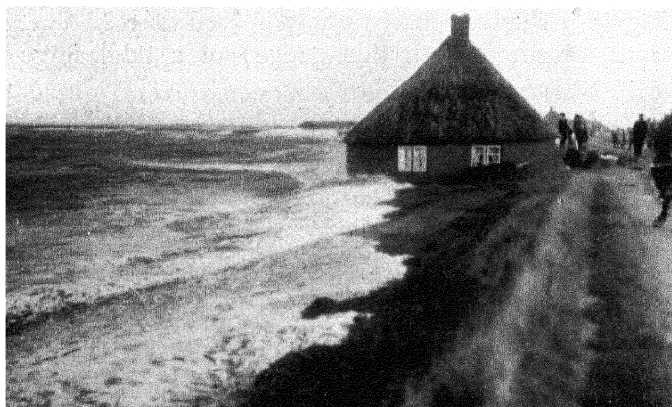
FIG. 4. Norderhafen on Nordstrand (northern Germany); tidal surge on October 18, 1936. The house, built on the dyke itself, was severely damaged. (Photograph: A. Busch, Morsumhafen.)
