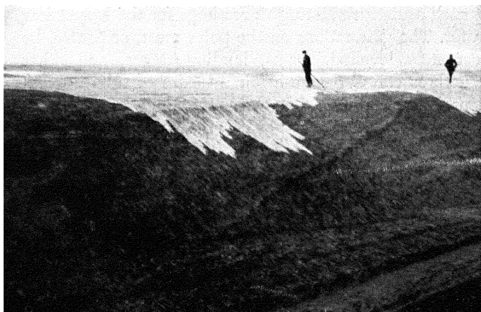
FIG. 6. Near Nordhafen on Nordstrand (scen from the roof of a stables on the marsh) on October 18, 1936. The high water has reached the dyke and is pouring over the top. (Photograph: A. Busch, Morsumhafen.)
