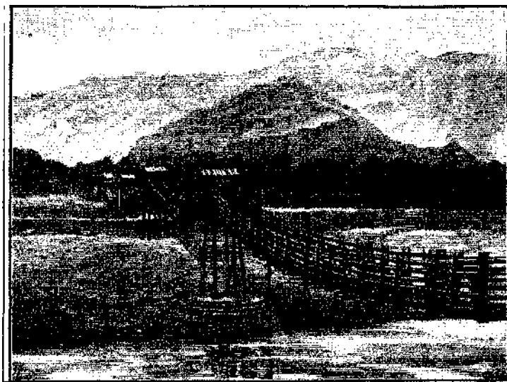
Bridge near Kwan-hsien (Ch'eng-tu).
