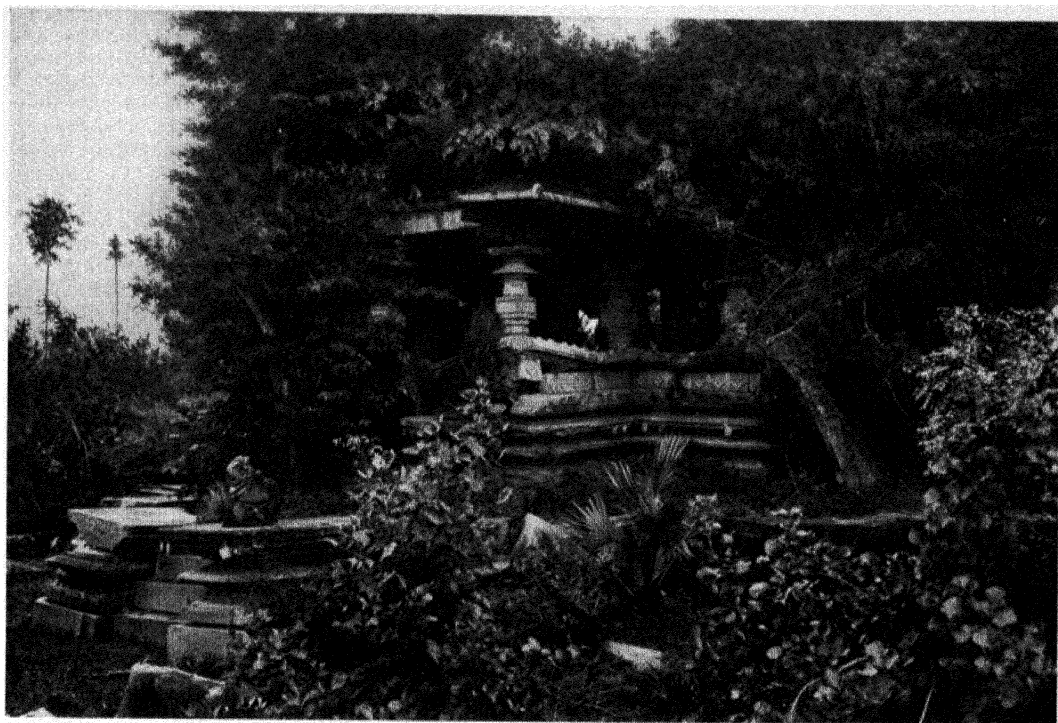
(a) A TEMPLE AT KATĀCHPŪR, WARANGAL DISTRICT: BEFORE RESTORATION
