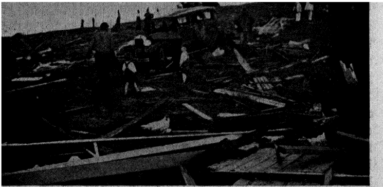
Fig. 78f. What Remains of Several Farm Buildings and Automobiles after the Tornado has Passed. Photos by Otto Wiederanders.
