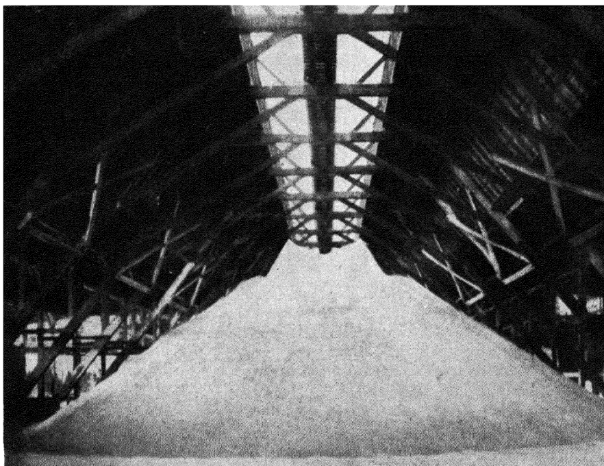
FIG. 72.—“A” FRAME BUILDING SHOWING PILE OF SUPERPHOSPHATE
