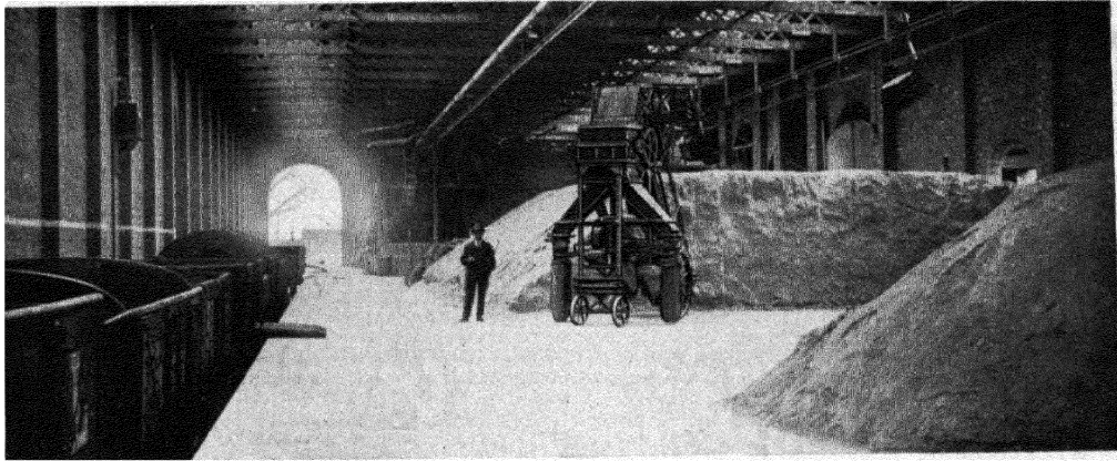
FIG. 74.—SUPERPHOSPHATE STORE BUILT IN BRICKWORK
