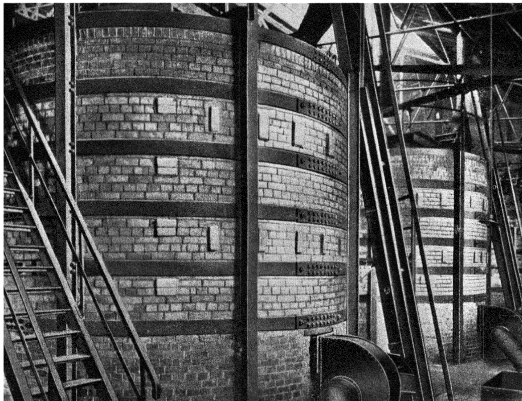
FIG. 151.—VIEW OF TWO HARRIS CIRCULAR SPENT OXIDE FURNACES
