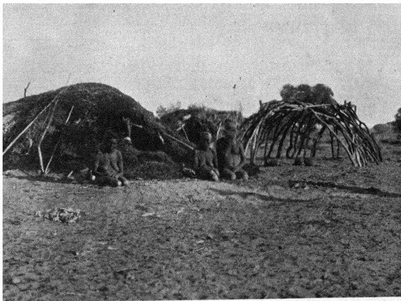
FIG. 16.— POONGA IN COURSE OF ERECTION.
