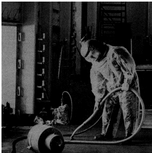
Figure 3. Pressurized suit worn in the active corridor between two rows of large glove boxes. The suit is protected by a disposable plastic overall
