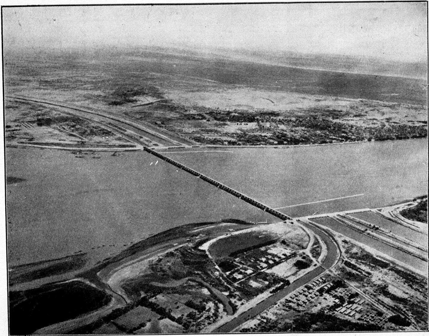
A general view of the Llyod Barrage and its seven canals.
