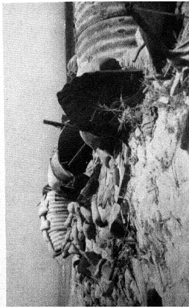
12. Typical sandbagged Anderson shelters before and after the Monte Bello explosion.
