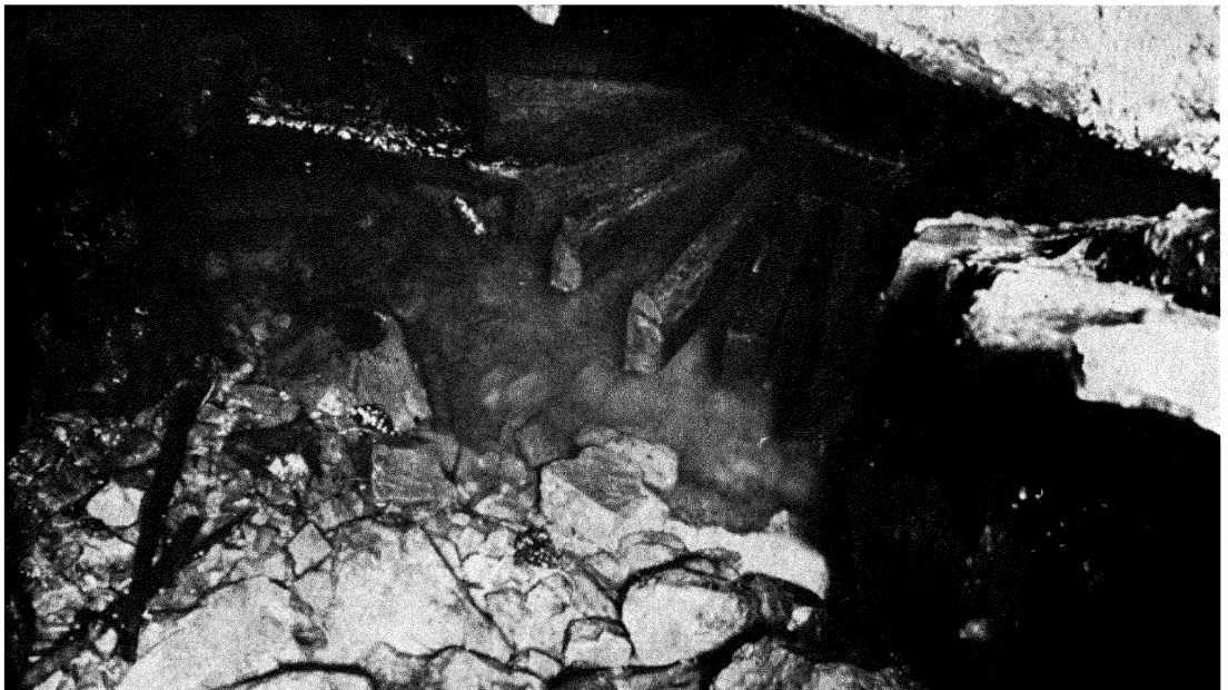
Plate 16. Turbine Water Mill. Rotor blades.
