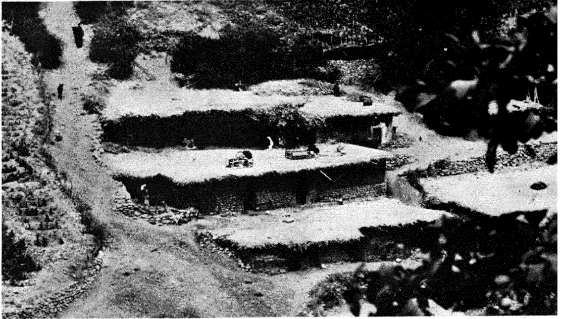
Plate 3. Dwellings. Typical house construction, Dergala.
