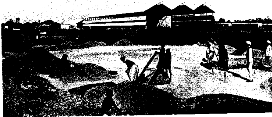
RAILWAY WORKSHOPS, GOYA GATE, JANUARY 1ST, 1922.
