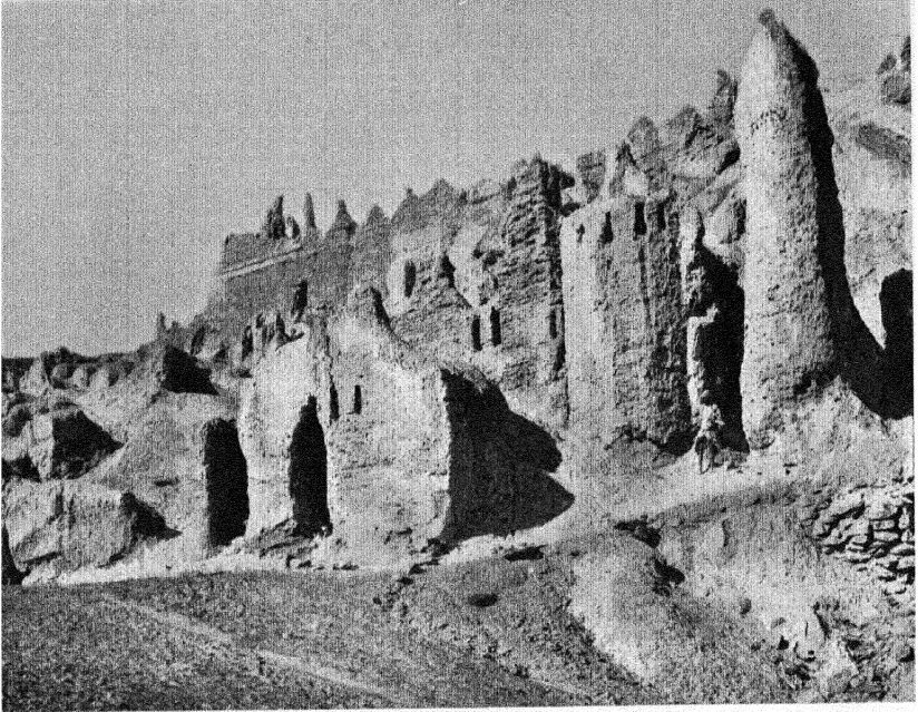
FIG. 31.—LOWER GATE AND TERRACES ON EAST SLOPE OF RUINED SITE, KOH-I-KHWAJA HILL, SEISTAN.
